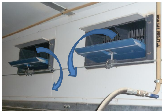
Low air speed. Cold air drops to the floor.
