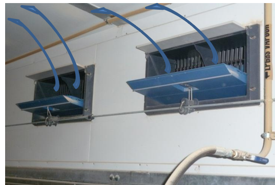
High air speed. Cold air mixes with hot air near ceiling.
